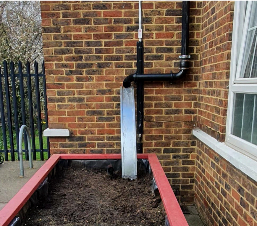
Figure 18: Finished installation of the water chute.
