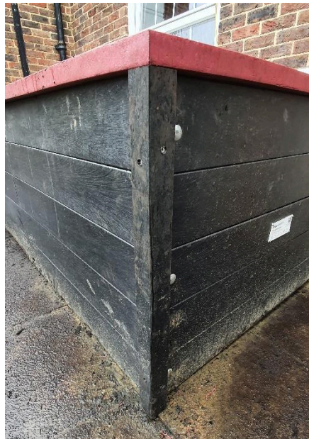
Figure 33: Screw positions on corner posts.
