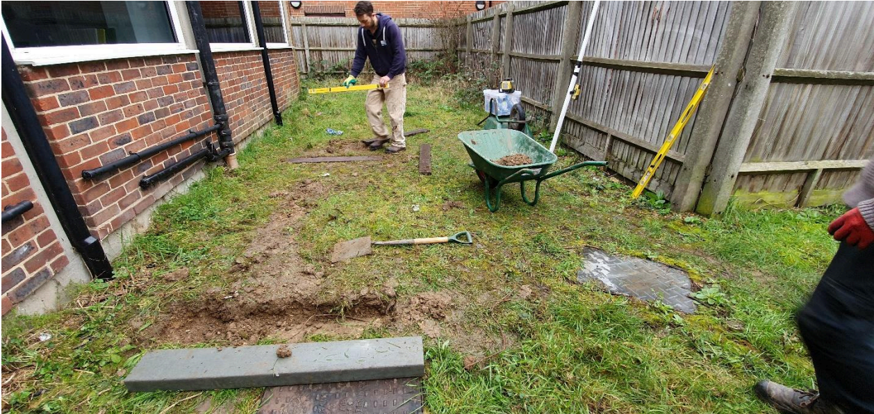
Figure 1: The ground being prepared for introducing supporting platforms.
