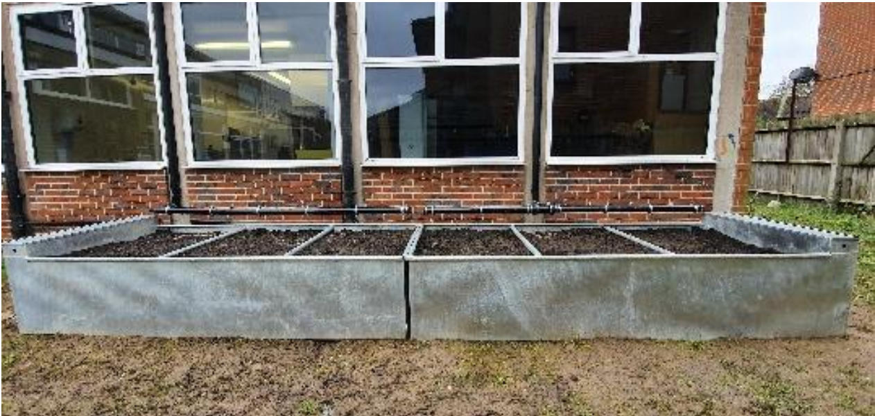
Figure 8.- Final look of the water trough planters. Note the changes in the configuration of the downpipe and the distribution pipes.
