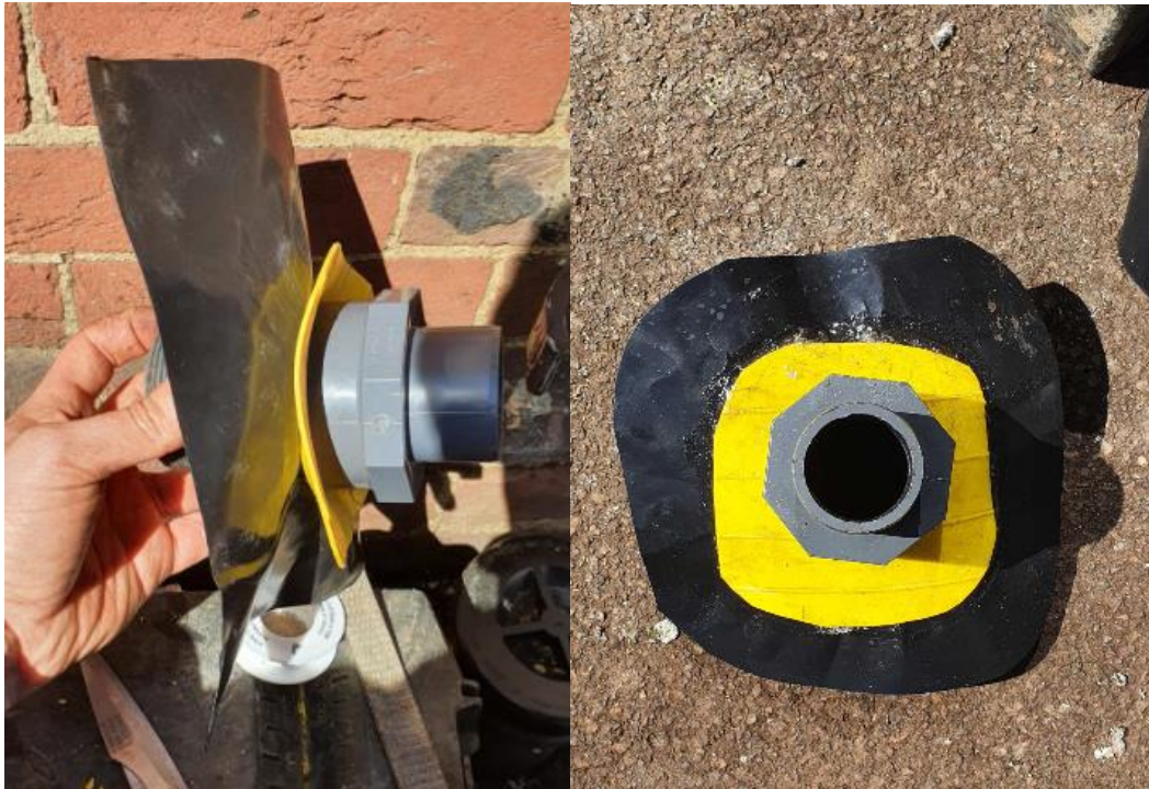
Figure 43: Improved method used to create a waterproof seal in the outflow.
