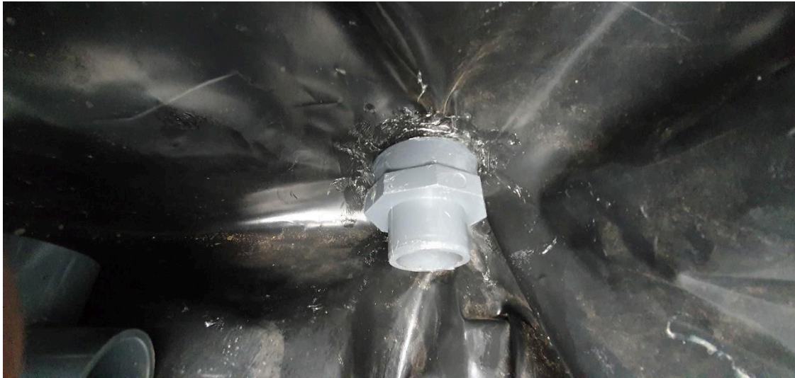
Figure 42: Inner section of the tank connector composed of a threaded nipple and two female adapters.
