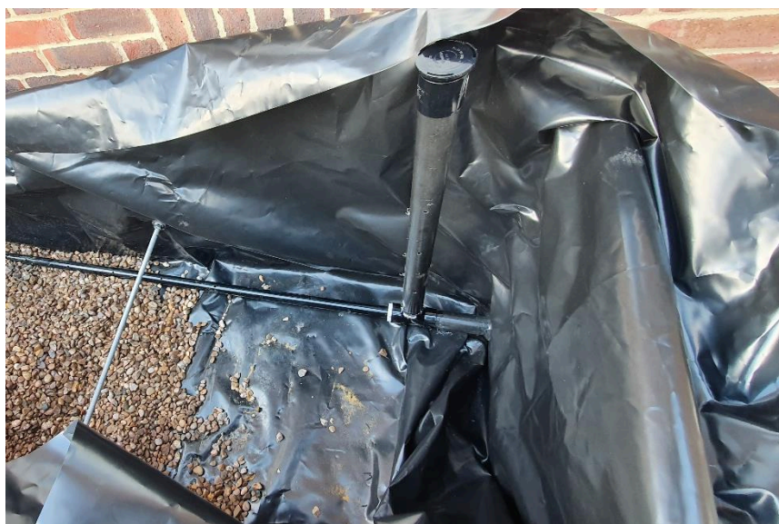
Figure 21: Introduction of gravel into the planter.
