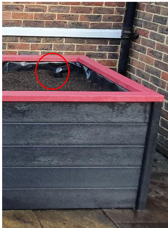
Figure 49: Elbow attachment in the overflow pipe to reduce the risk of blockages.
