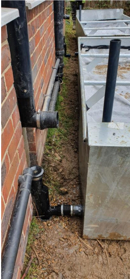
Figure 5: Water trough connected to the drain.
