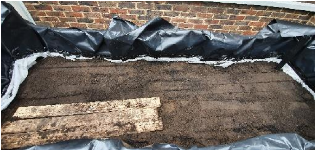
Figure 24: Soil being compacted using long wooden planks.
