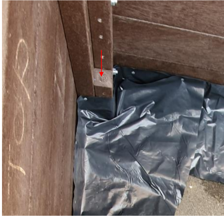
Figure 30: Installed piece securing the leg extensions to increase the planter stability.
