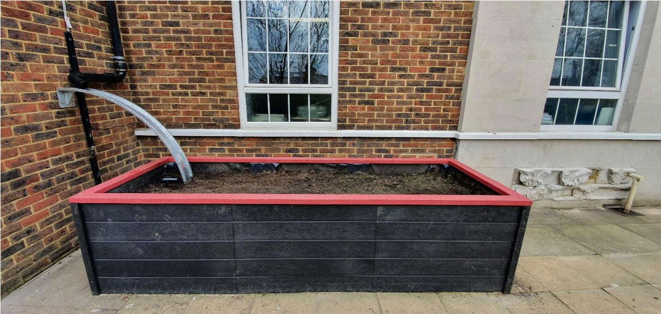
Figure 17: Finished installation of the water chute.
