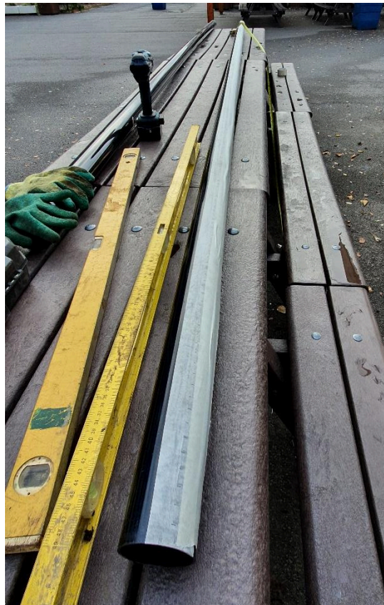
Figure 10: Marked masking tape in a straight line on the pipe before being drilled.
