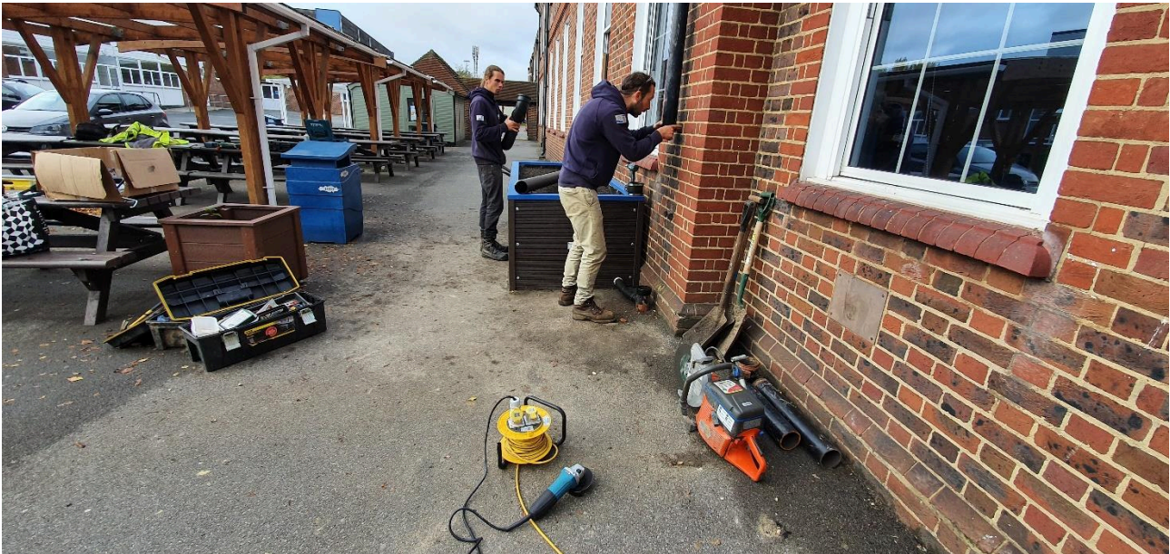
Figure 11: Downpipe being cut after checking the position of the fittings.
