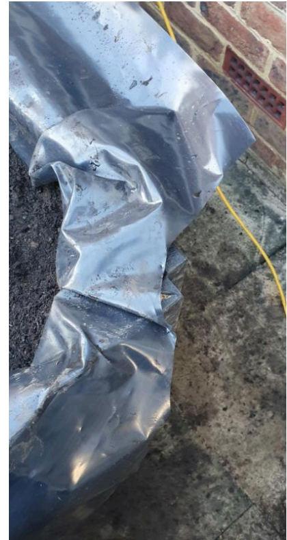
Figure 45: In this image, excessive folds and HDPM material in the corner have been removed.
