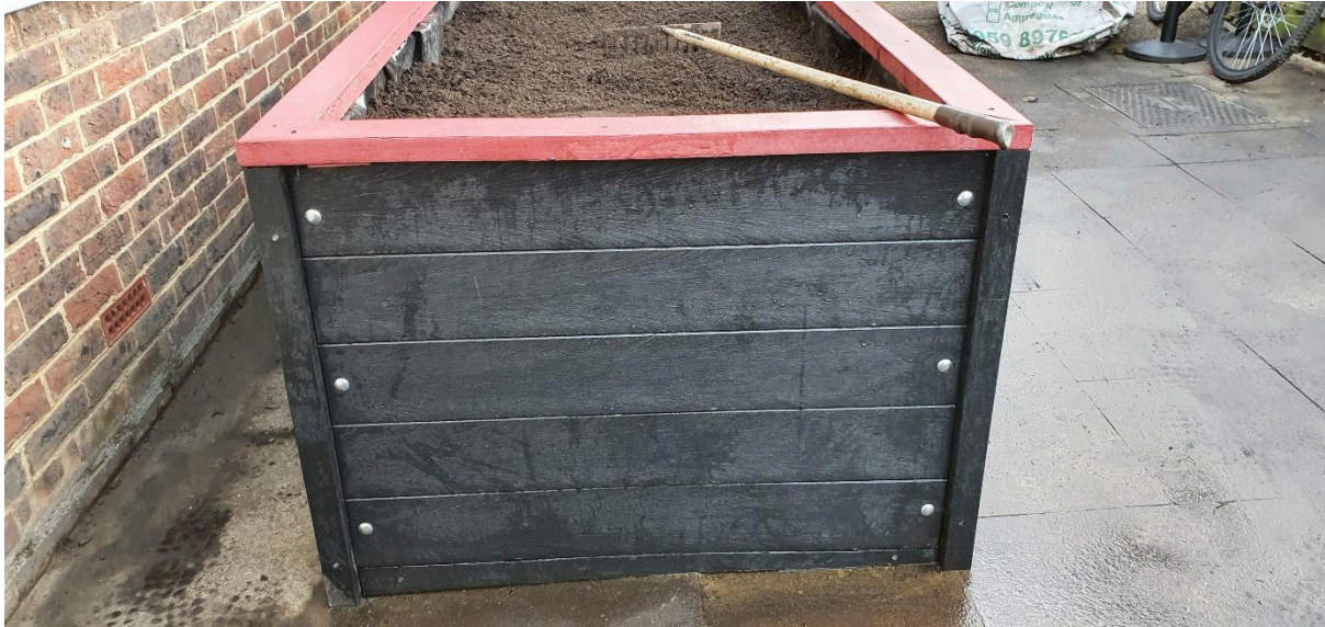
Figure 40: Final look of the planter. Note how the bottom section is covering the gap created when modifying the planter's height.
