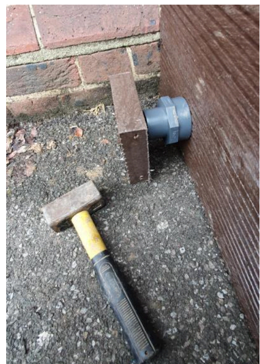
Figure 44: Introducing the tank connector on the planter. This process has to be done carefully to avoid any damage in the fitting.
