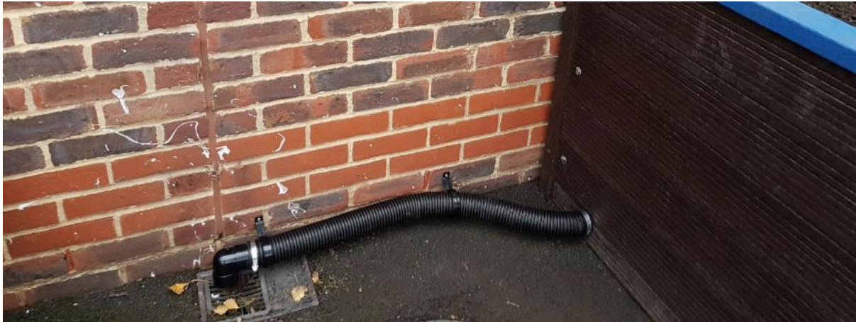
Figure 5. Example of connection back into existing drainage
