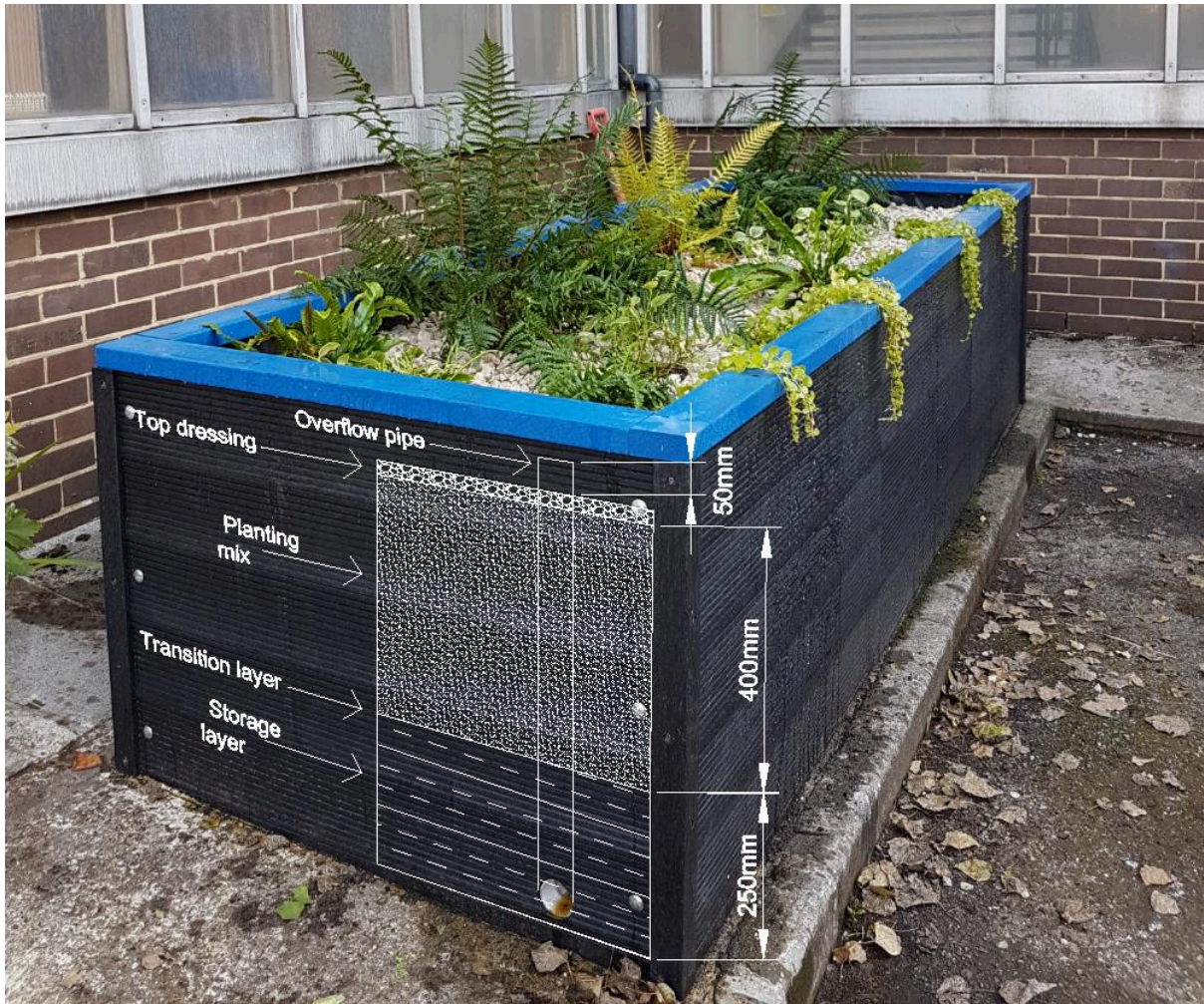
Figure 1. Completed planter, with illustration of internal planting layers. In this example, geocellular crates were used as a sub-base/drainage layer.
