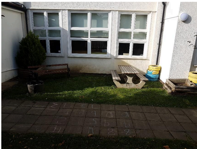
Figure 2. An area too close to the school building.
