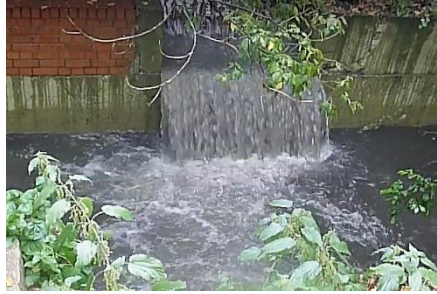
Epsom Storm Tanks (Photo thanks to SERT)
