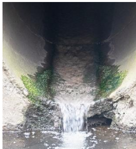
NM Railway Bridge
