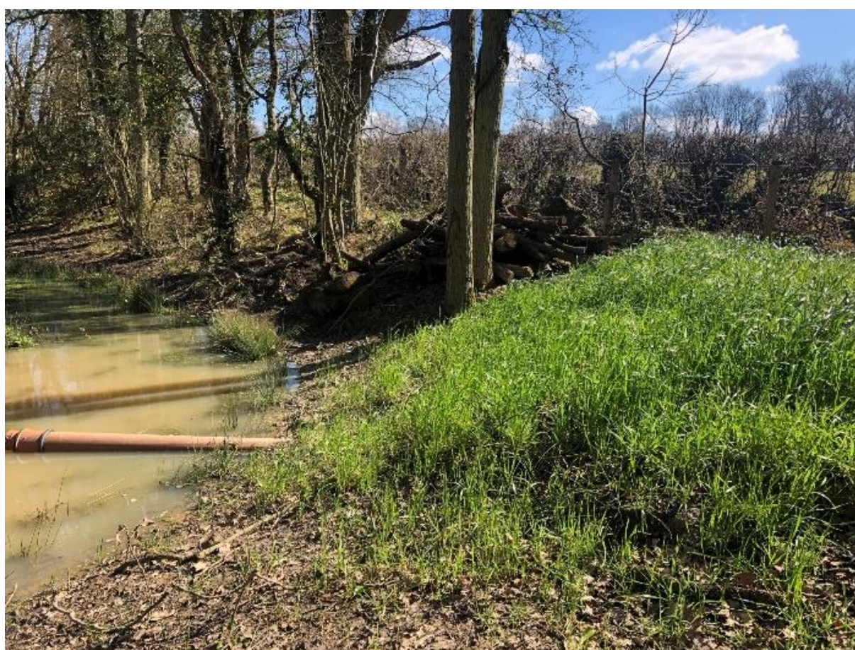
Figure 83. Sowing seed mix was successful in vegetating the pond's bund to make it less likely to be eroded.
