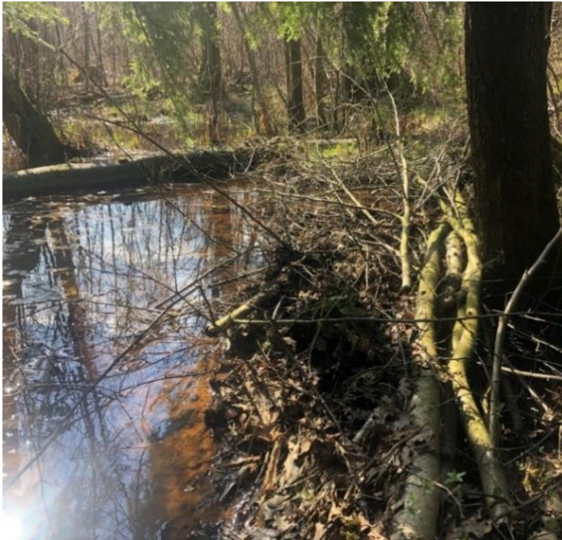
Figure 28. Photo showing the build-up of woody material, leaf litter and silt upstream of a LWS in Bedgebury Forest
