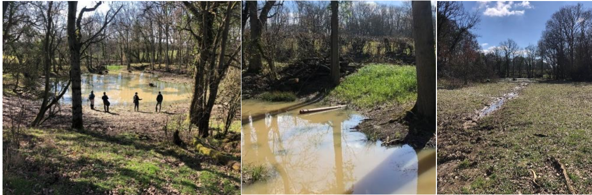
Figure 72. Kingsnood pond one year after installation (left). The bund and pipe maintain the desired water level (centre). Offtake channel from main river to the pond (right).
