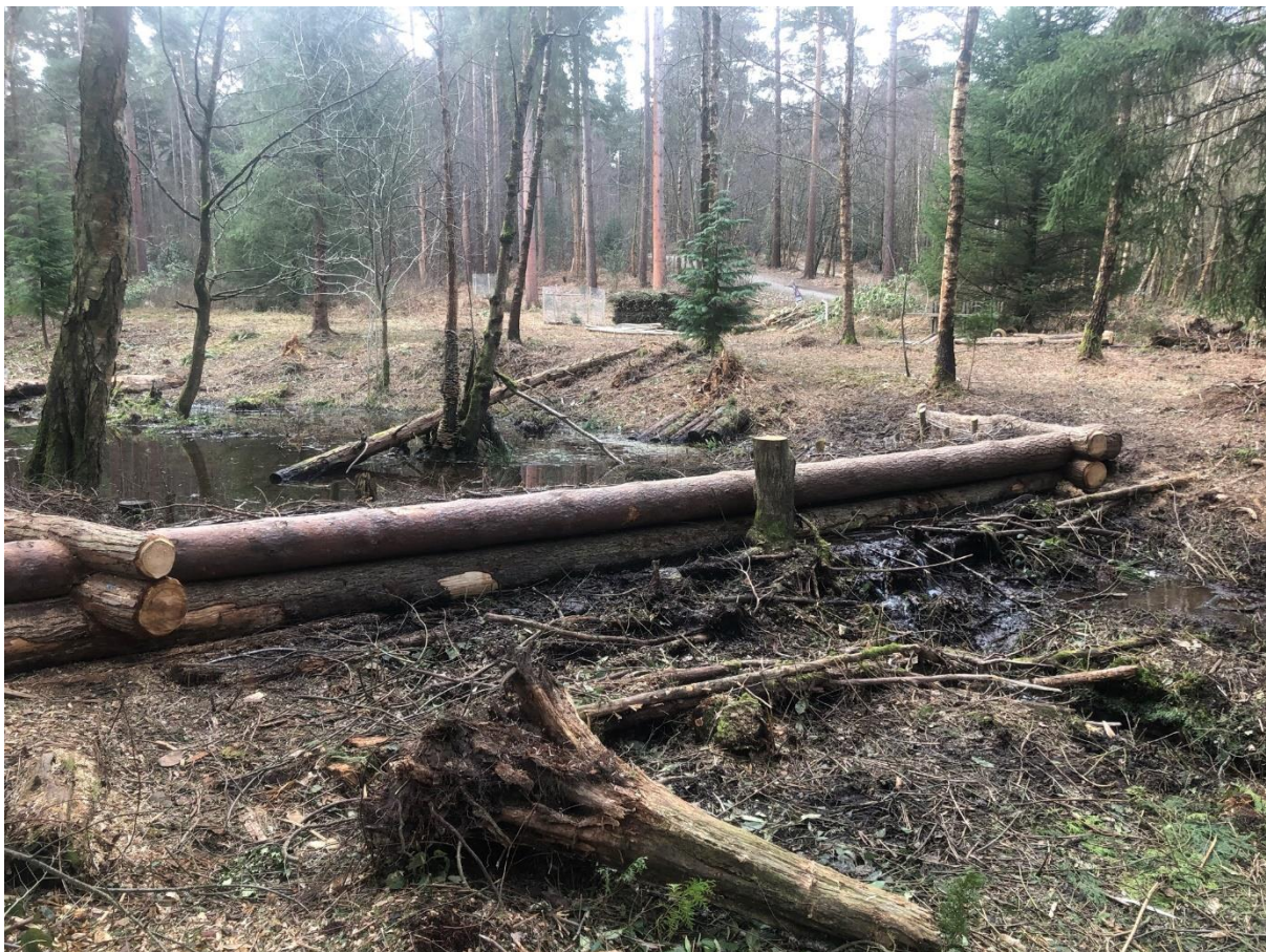
Figure 26. The largest and most downstream of the series of 4 demonstration LWSs installed at Bedgebury Pinetum, alongside paths that experience a high footfall.
