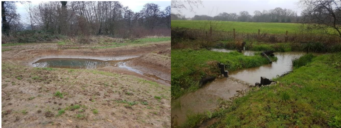
Figure 16. Off-take channel corner pond (left), and control structures (right)
