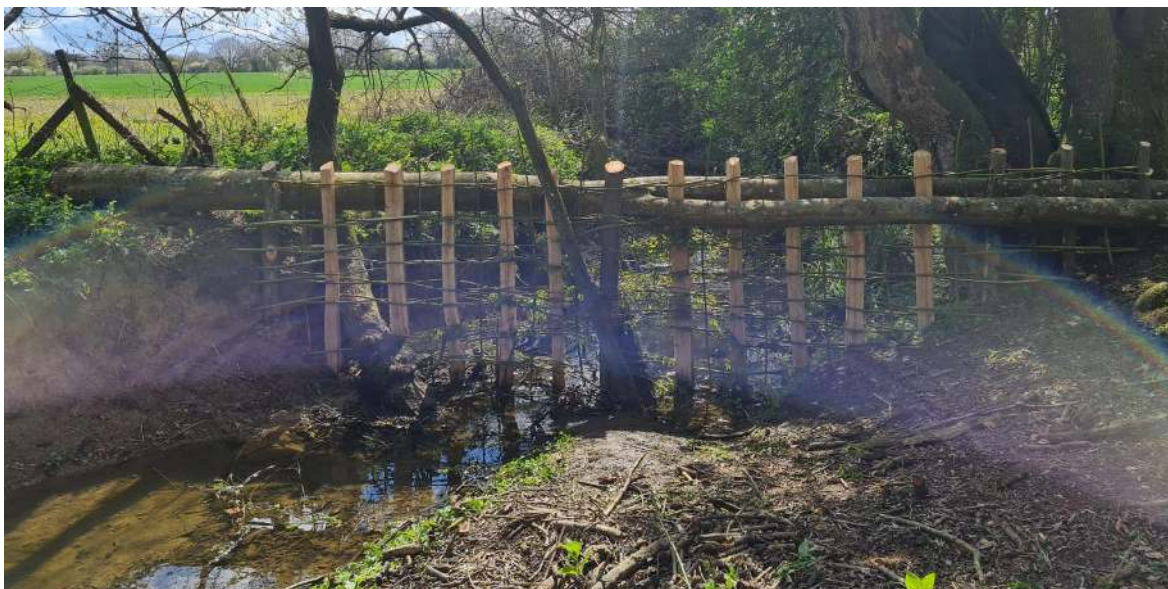
Figure 73. Willow was weaved through a LWS on Boy Court Farm, adapting LWS function to capture silt and offer maximum benefits to the specific site.
