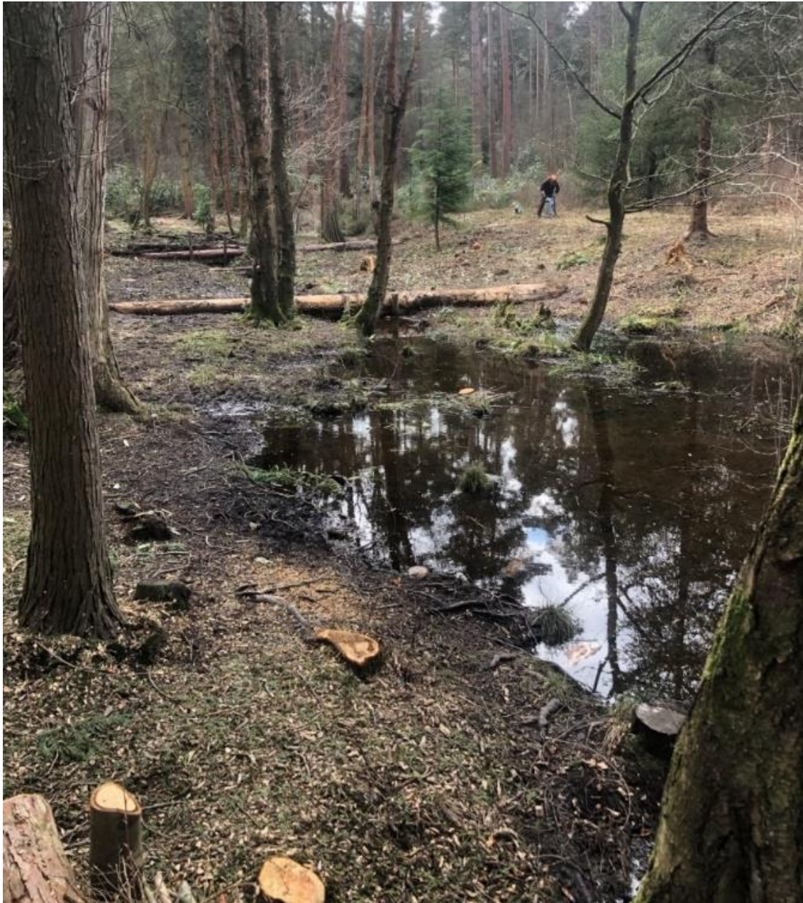
Figure 33. Contractor (far bank) can be seen moving a large, felled tree using only winches. On the near side of the bank, there has been minimal disruption to the soil and riverbank as trees have been felled and moved using low-impact methods.
