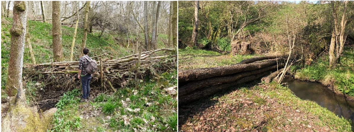
Figure 51. LWSs installed in Church Wood (left) and across the wider floodplain on the main river running through the valley at Milrough Wood (right)
