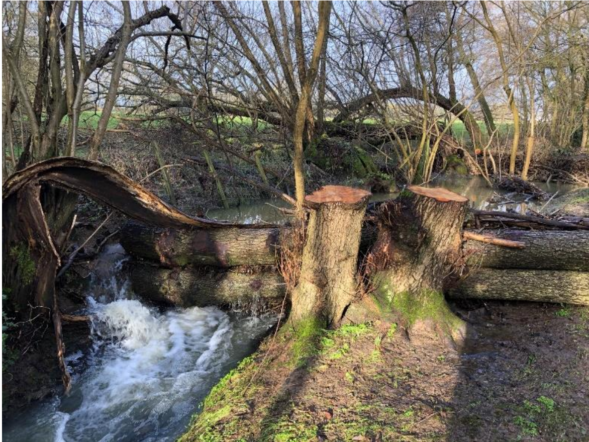
Figure 75. LWS at Stonehall Farm after a rainfall event, visibly holding back large quantities of water and slowing the flow.
