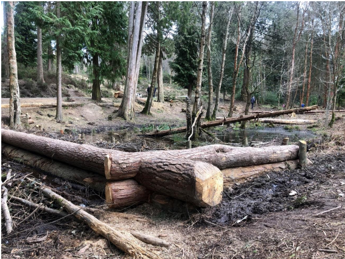
Figure 31. The series of 4 large demonstration LWSs were located alongside a path (running along the watercourse from the left of the photo) in the well-visited Pinetum.
