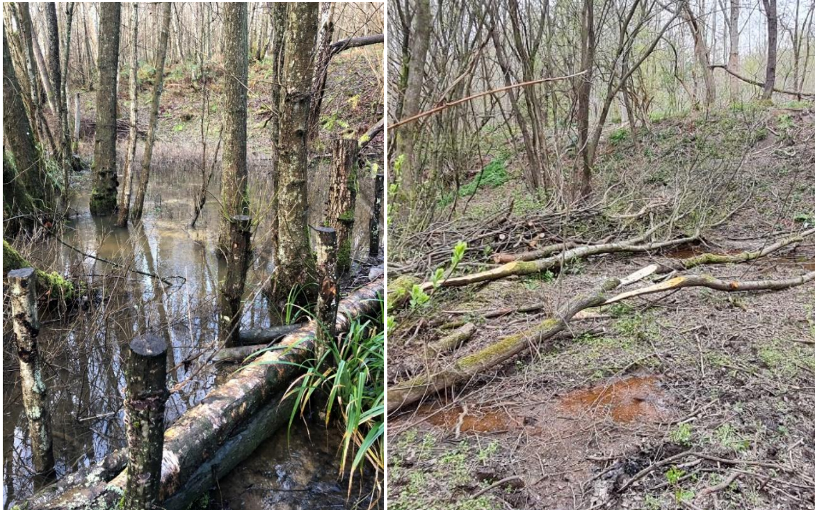
Figure 57. Regenerative LWS design: willow stakes, used to secure LWSs, have taken root and that the LWS is starting to regenerate, as shown by their new shoots (left). LWSs include hinged trees (right).
