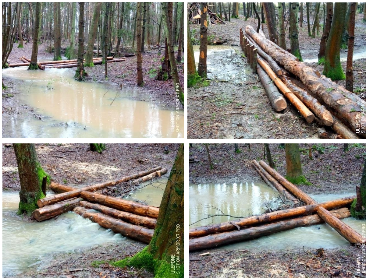
Figure 74. LWSs in Birch Wood in a flood event. A higher water level is clearly visible upstream of the LWS and debris collected is also visible, improving the water quality.
