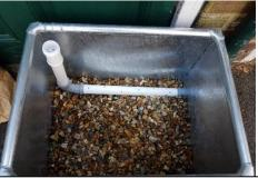
The gravel can be used to prop up one end of the base drainage pipe so it slopes slightly towards the outlet. Keep adding gravel until the pipe is just covered.
