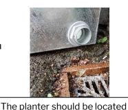
so it drains to the existing drain
