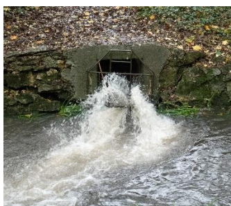
Ewell Storm Tanks
